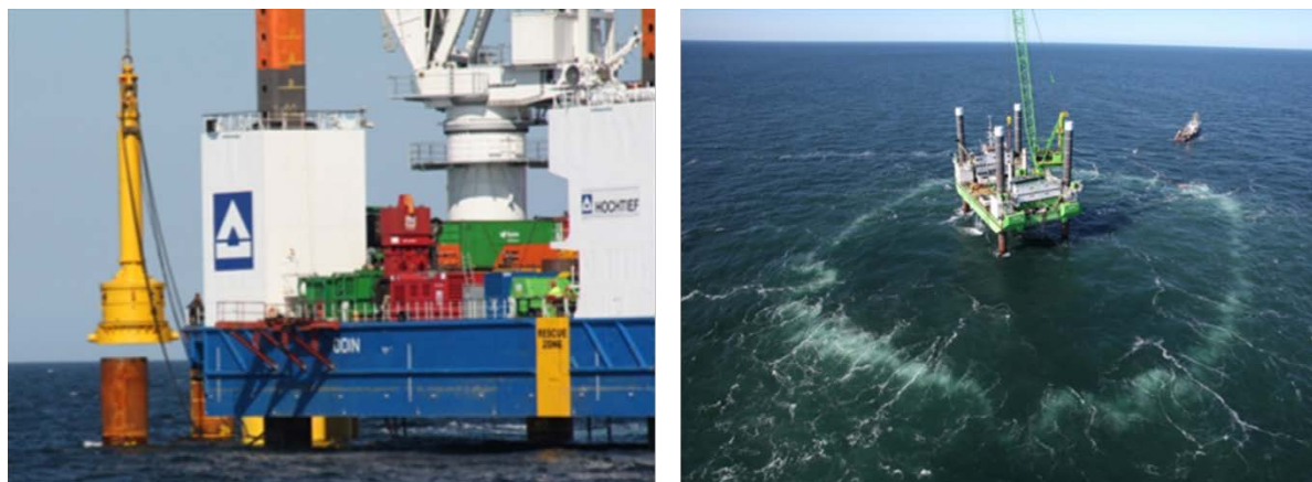
Fig. 11: Bubble curtains minimise underwater noise from pile driving for wind turbine foundations (left: photo Klaus Betke; right: photo Trianel).
