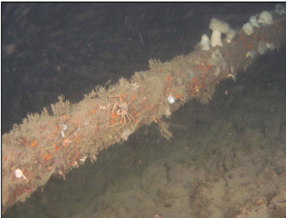
Fig. 50 Subsea power cable, in place for approximately 50 years, covered with sessile encrusting organisms at Vancouver Island (BCTC 2006).
