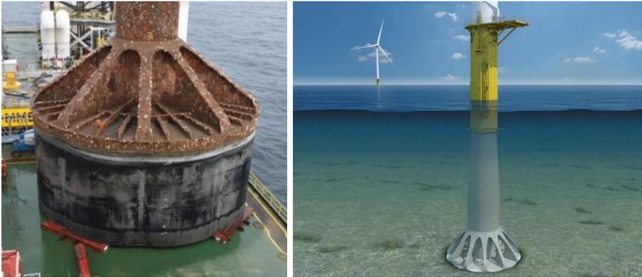
Fig. 14. Installation of a Mono Bucket after full decommissioning (left). Design of a Mono Bucket carrying a wind turbine (right) , ©Universal Foundation.
