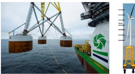
Fig. 13. Installation of a suction bucket jacket (left, OWF Borkum Riffgrund 2, © Ørsted). Idealised SBJ loading (right, OWF Borkum Riffgrund 1, Ørsted (2019)).
