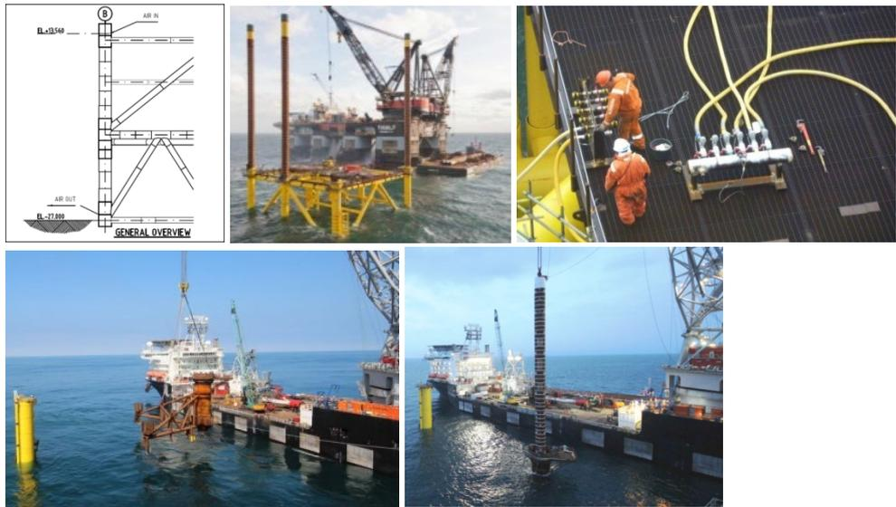
Fig. 5. Schematic drawing (top left) and application of jacket legs extending above the water surface and thus acting as cofferdams at Dolwin alpha (top middle); air hoses for dewatering the pile sleeve (top right) at DolWin alpha; Installation of a cofferdam extension on top of the pile sleeve (bottom left) and piling through the complete cofferdam at BorWin beta (bottom right) © TenneT
