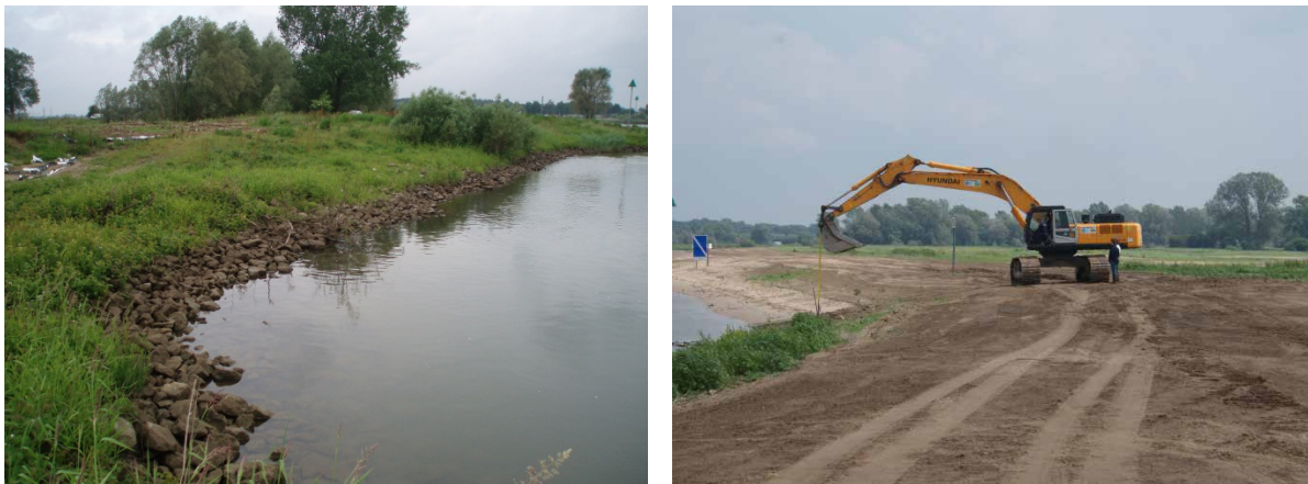
Abb. 24: Restoration of river banks to comply with the Water Framework Directive, before (left) and after (right).
